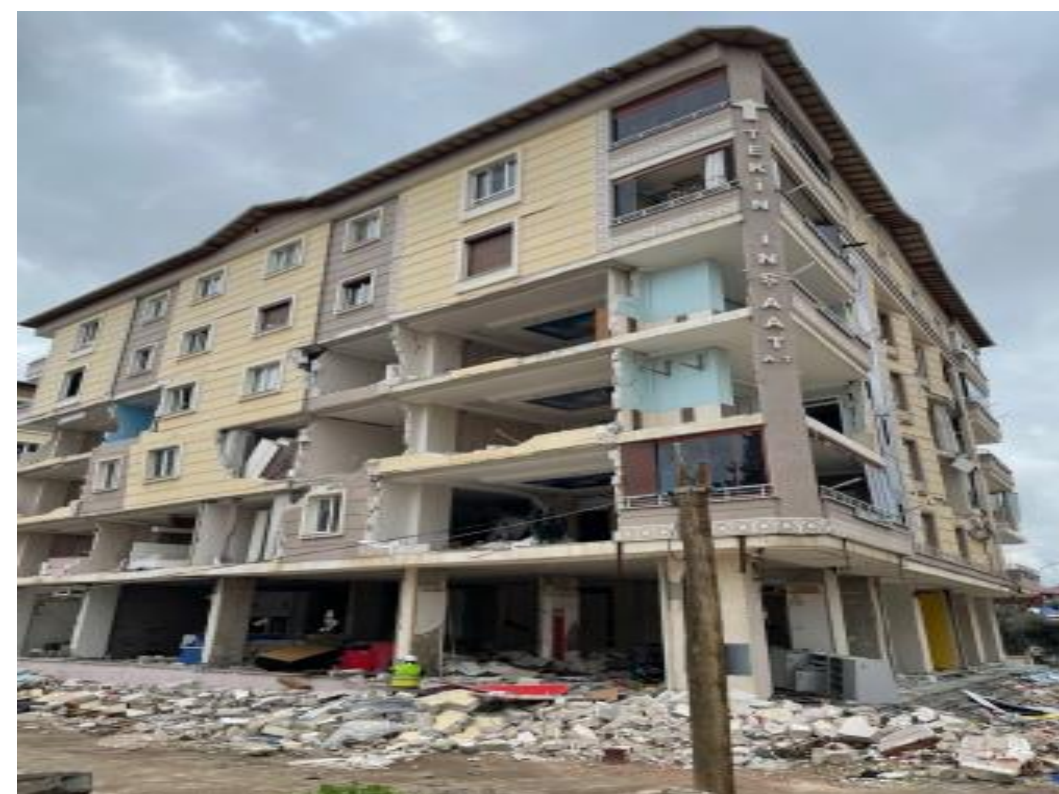
Figure 2- Non-structural damage in the envelopes of a residential building in Turkey (6 th February 2023) [4]
